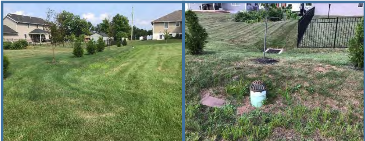
Detention Berm - BMP #20B1 Photos taken during 2021 inspection.
